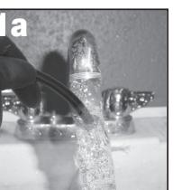
**Do:** Place end of hose under hot tap water for 1 minute. This will soften the hose and help insure the hose is pushed all the way down to the flange.
